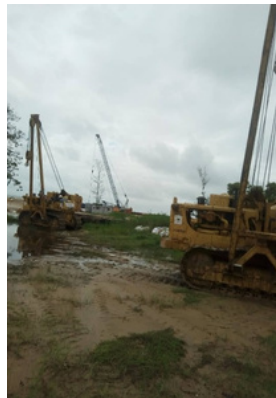
36" Pipe-Laying For Dangote Fertilizer
