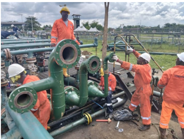
Re-routing of Flowline and Installation of Multi-phase Flow meter – NEPL
