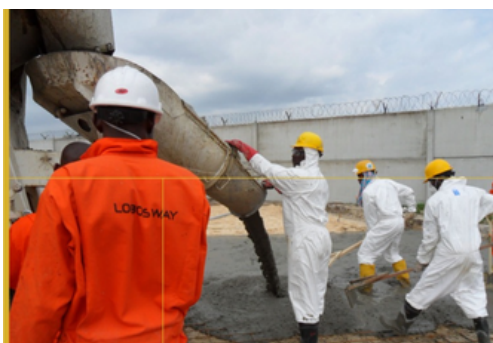
Site Preparation For SAPIEM, NPA Warri (SSAGS Project)
